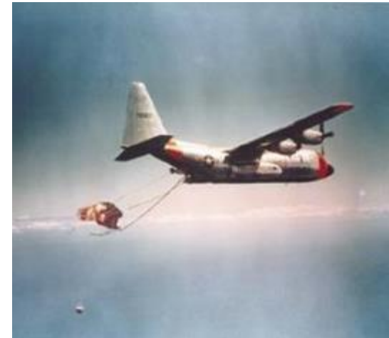
JC-130 recovery aircraft, U.S. Air Force retrieves a Corona satellite film-return capsule, using a "bucket," over the Pacific.
